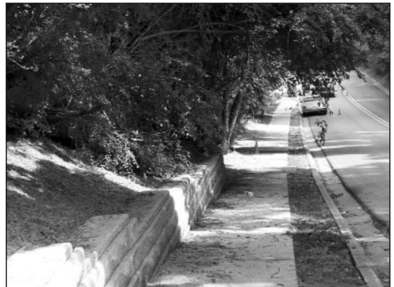
Installation of the Foster Street sidewalk was funded with CDBG money.
