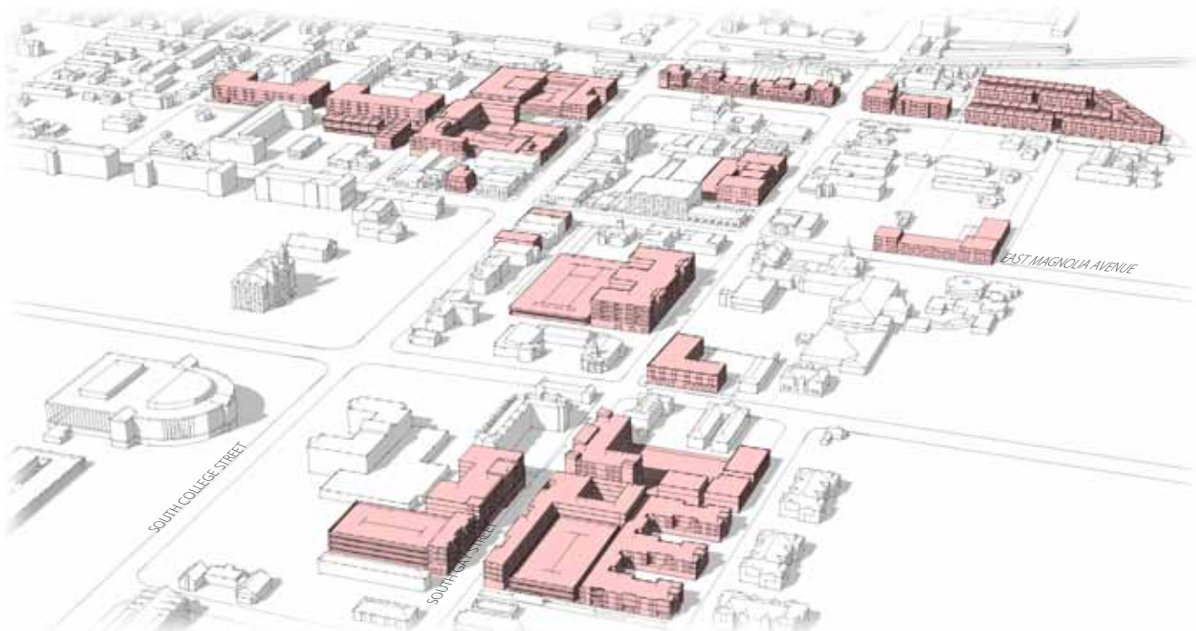
Bird's eye view looking NW
