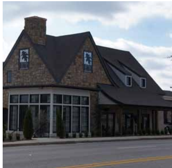
New development near intersection of E. Glenn & N. Gay.
