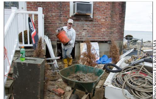
Joe Barry, a volunteer from the United Methodist Committee on Relief, helps a homeowner clean after Hurricane Sandy washed away exterior walls and completely filled the basement.
